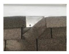
**NOMINAL REPAIR:** Some of the sewer vent pipe boots are top-nailed and have exposed nail heads. See example in photo.
