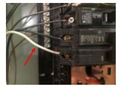
**MINOR REPAIR:** The mini split heat pump is labeled for a maximum of a 20-amp size breaker. It is presently "protected" by a 30 amp breaker. In the
